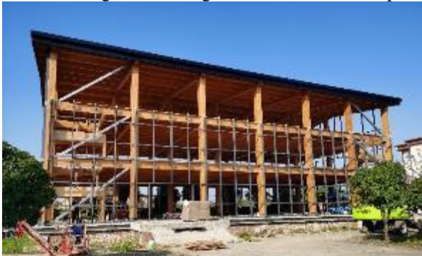
(a) laminated bamboo office building with 1,500 square meters
