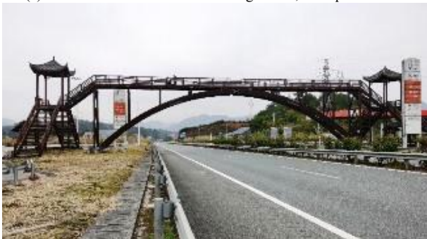
(b) glued-laminated wood footbridge with 39.5 meters
